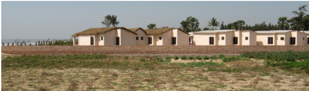
Construction On Beach Flattening Sand Dunes
